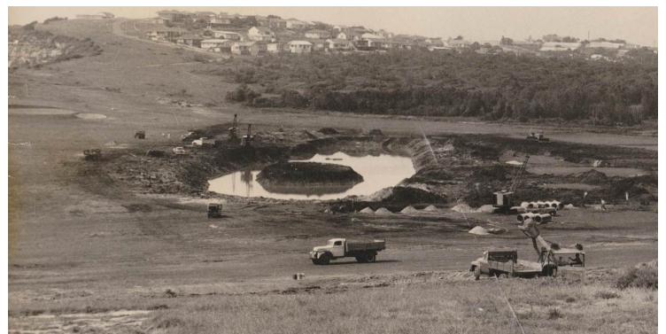
Course construction at Mona Vale. 4
